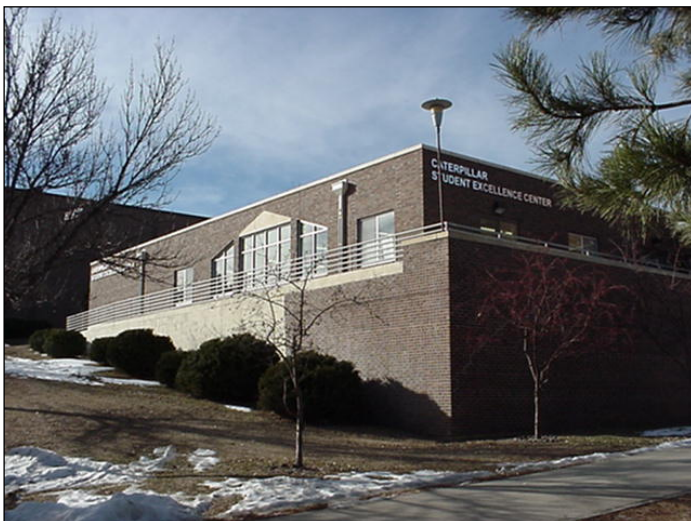
Photo Four Caterpillar Student Excellence Center
